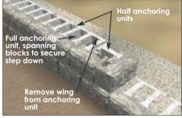
Install the half of an anchoring unit.
