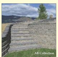
Allan Block's patented front lip provides a built-in edging that not only works with Allan Block Capstones but also with pavers, poured concrete, crushed rock, mulches and flagstones. Ensure stair treads are secured in place for safe use. In colder climates, salt **CANNOT** be used on the blocks or AB Capstones as it will cause them to deteriorate.
