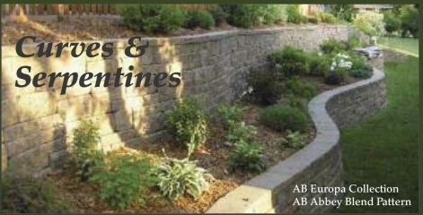
Flowing inside curves are achieved by a consistent spacing between the backs of the blocks as you build.
